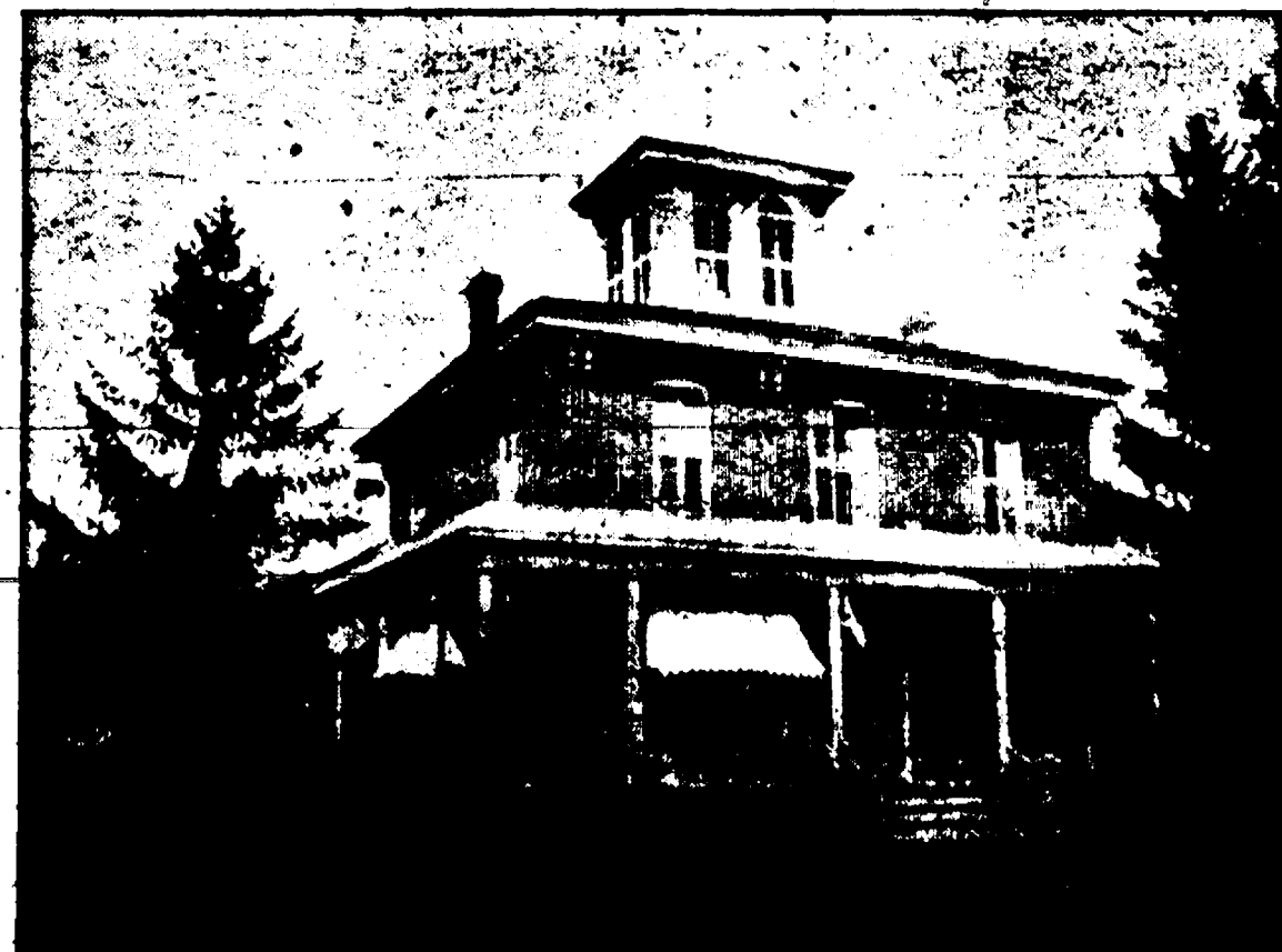
RESIDENCE OF J. J. TEEPLE.
