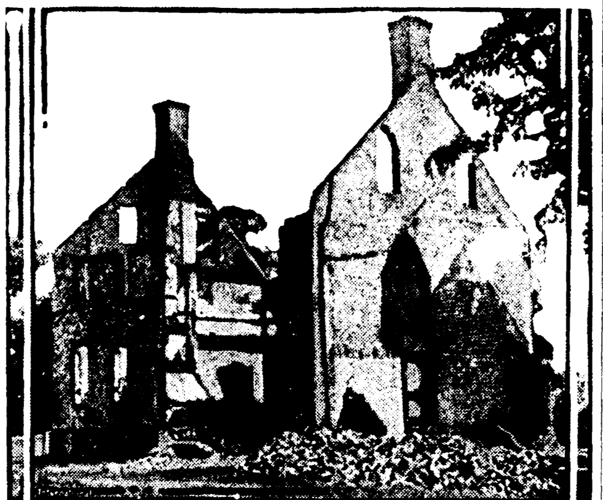
This photograph shows the ruins of the only house built by George Washington. It is situated at Hayfield farms, six miles south of Alexandria, Va. This building was constructed by Washington in 1765. About ten years ago the place was burned, only the walls remaining. The property was purchased by George T. Penny, who is to erect a modern home on the site. But the Daughters of the American Revolution are to place a marker at the gate, giving the history of the house.
